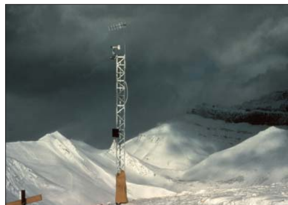
Meteorological conditions measured at Lake Louise, Alberta, Canada are telemetered via phone-to-RF link to a base station.
